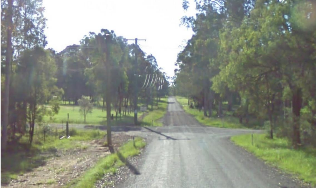
Figure 2-6 : View along Kerlew Street in the westbound direction
