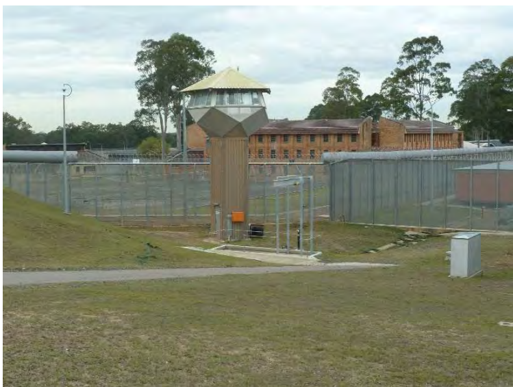
Figure 4 Existing medium security facility
