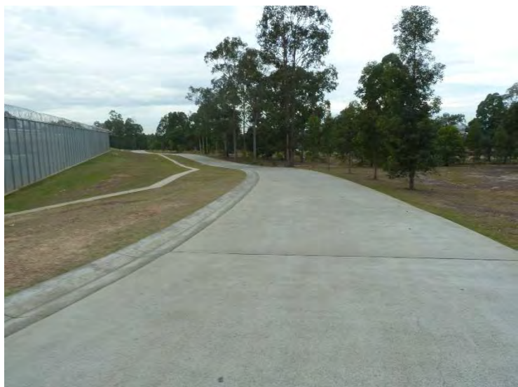
Figure 7 Existing main road to western gatehouse and car park
